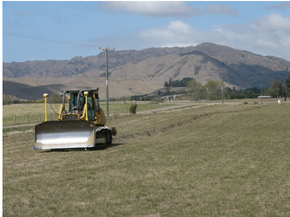
Ripping 700mm deep. 'One down, 1598 to go!'
