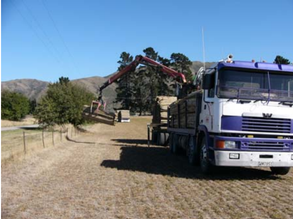
One of 50 truck and trailer loads of posts arriving!
