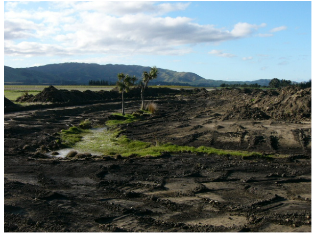
Old creek channels stripped of topsoil prior to drainage pipe being installed. Cabbage trees will be transplanted and then channel filled. Topsoil will be spread over fill.
