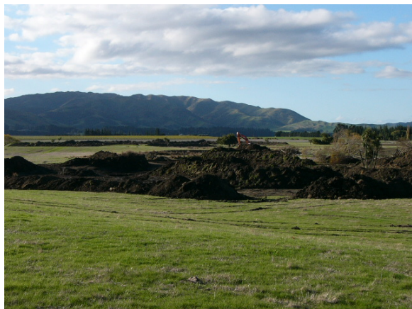
During topsoil removal 12/5/08
