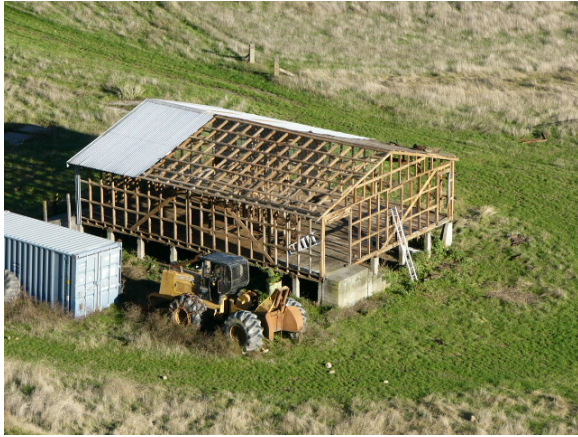
Iron being recovered prior to dismantling sheds
