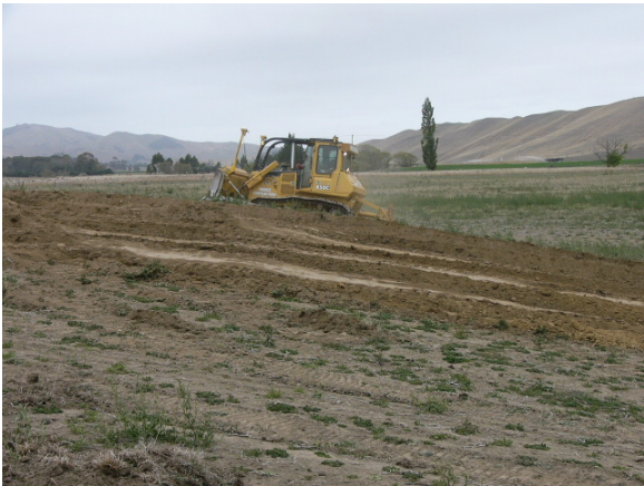
Contouring side slopes 'Marama Block'
