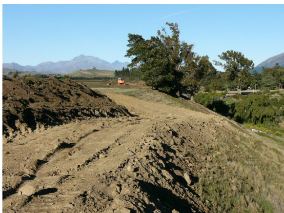
Benching of terrace edges prior to back filling
